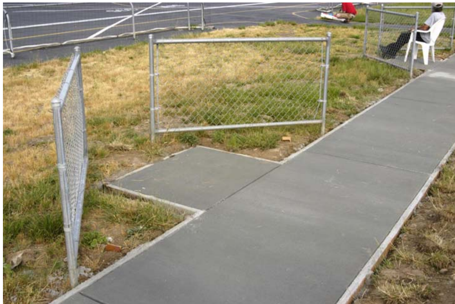
New concrete walkways and pads. Michael Luvara photo.
